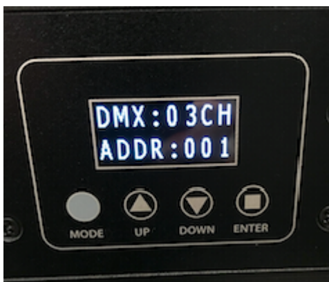
DMX CABLE CONNECTED
